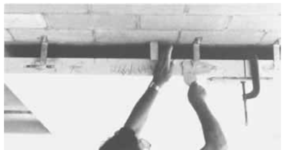
Lateral Adjusting Plate with S.S. Bar, Field Weld Plate to Angle
